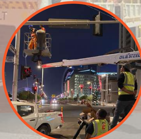
STREET LIGHTS REPAIRS AND MAINTENANCE
