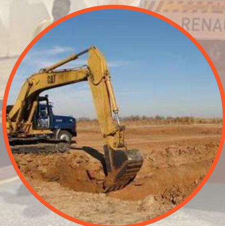
CLEARING OF CONSTRUCTION SITE
